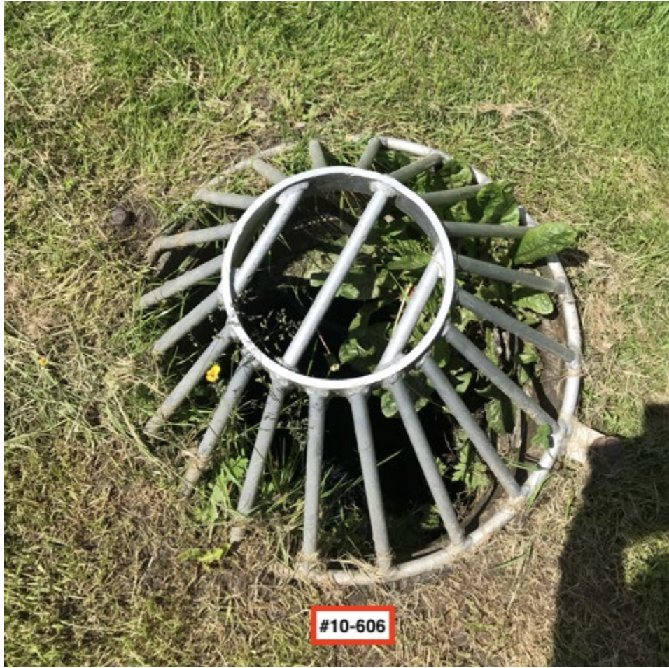
Close up of catch basin #10-606.
