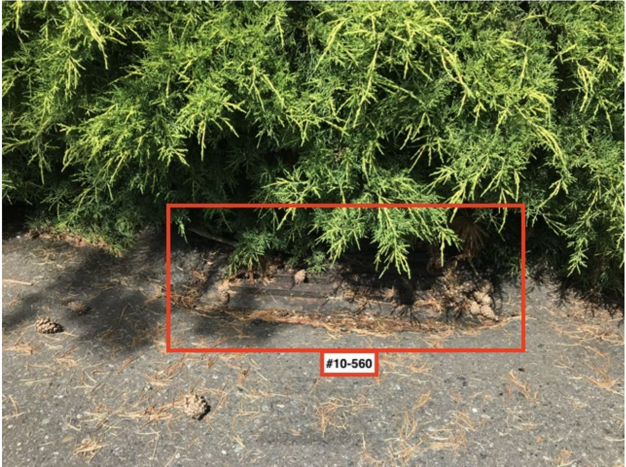
Close up of catch basin #10-560.
