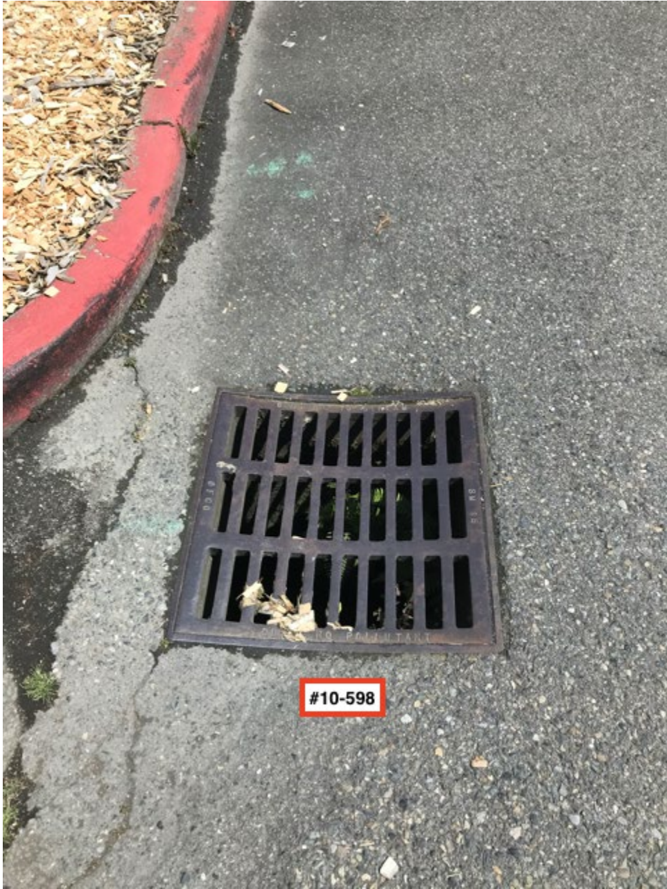
Close up of catch basin #10-598.
