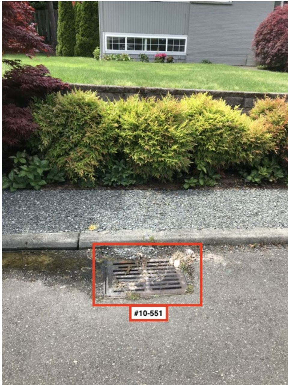
Facing W on 77th Ave SE, catch basin #10-551 in foreground.
