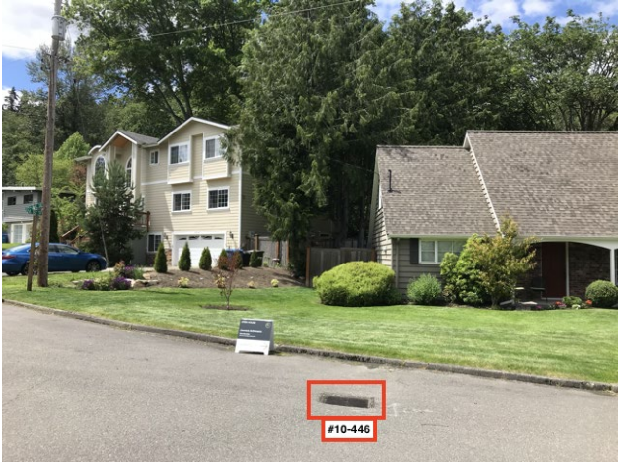
Facing W on 77th Ave SE, catch basin #10-446 in foreground.
