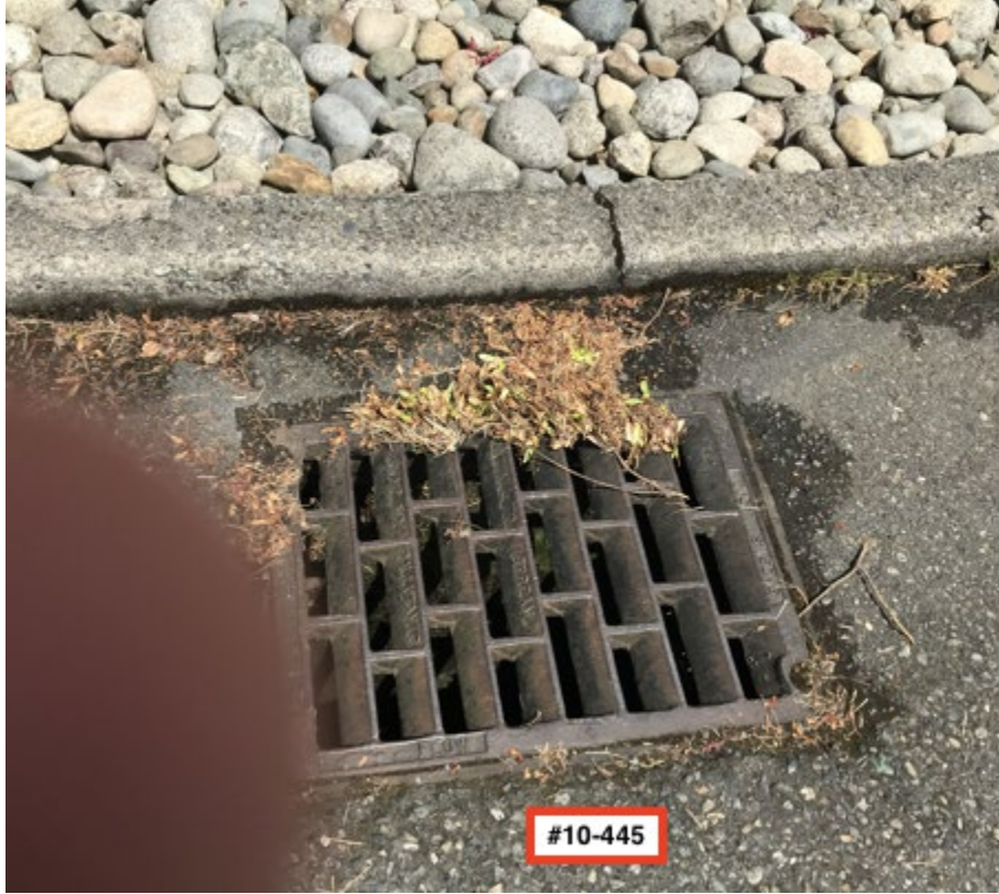
Close up of catch basin #10-445.
