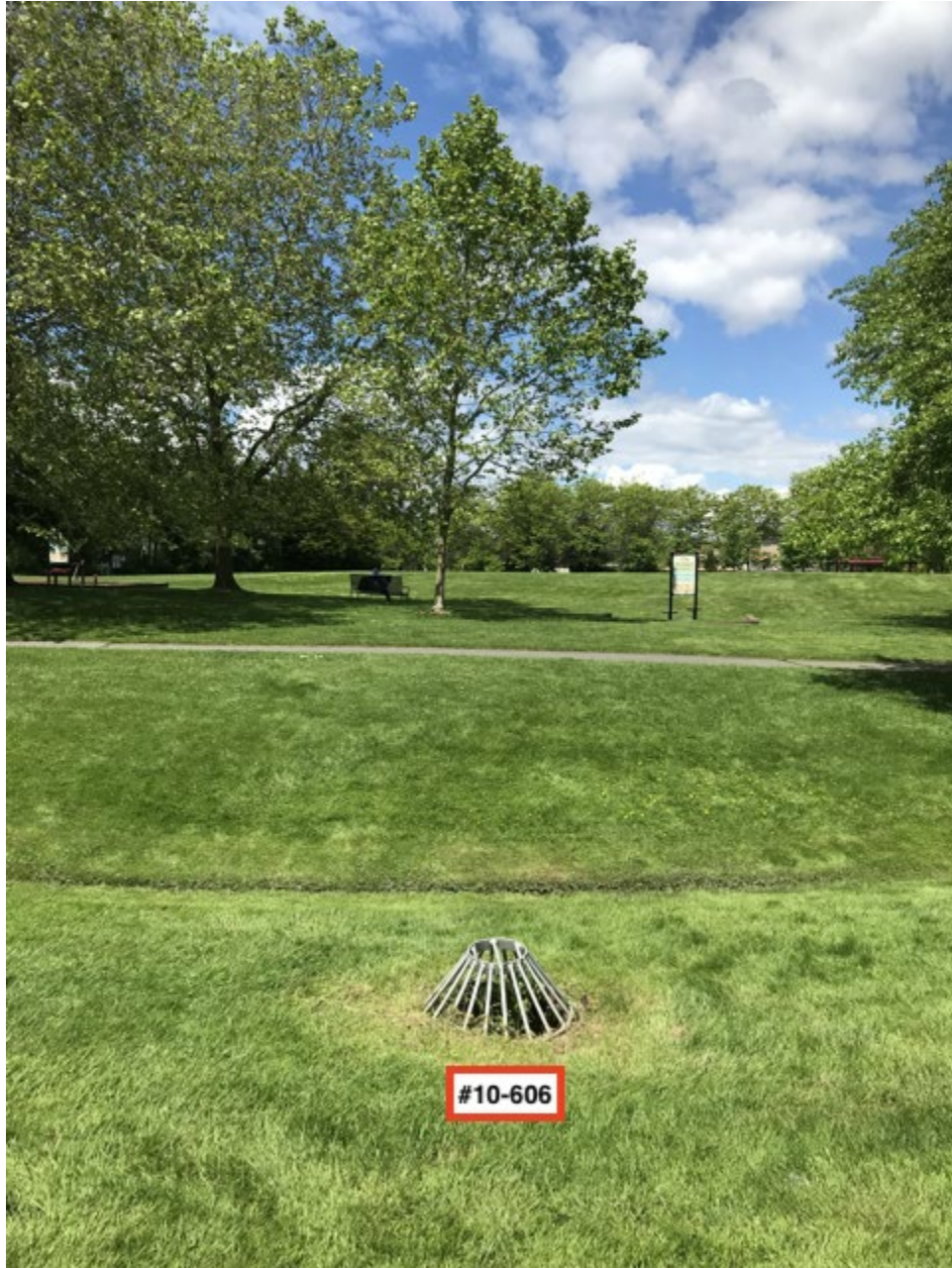
Facing N, with catch basin #10-606 in foreground.
