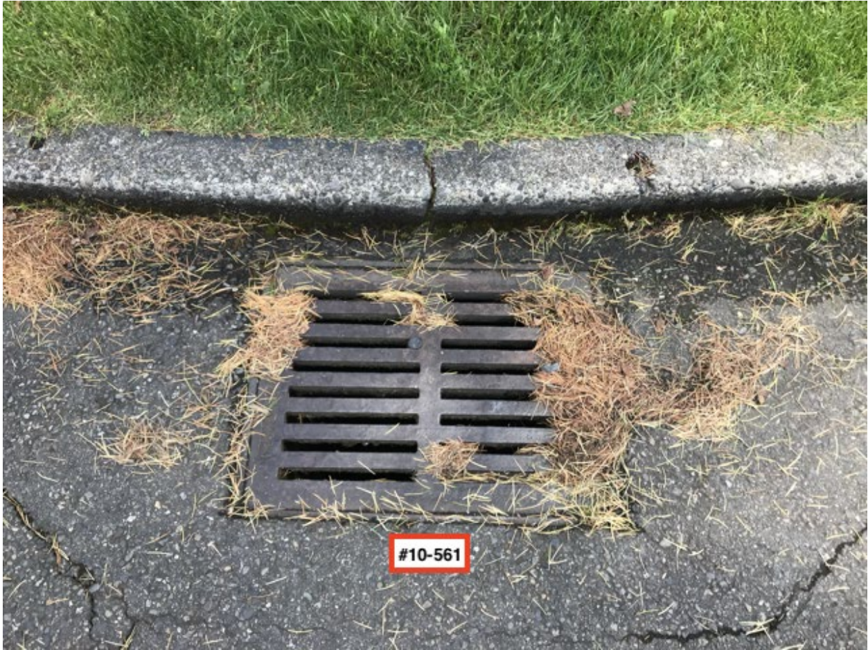
Close up of catch basin #10-561.
