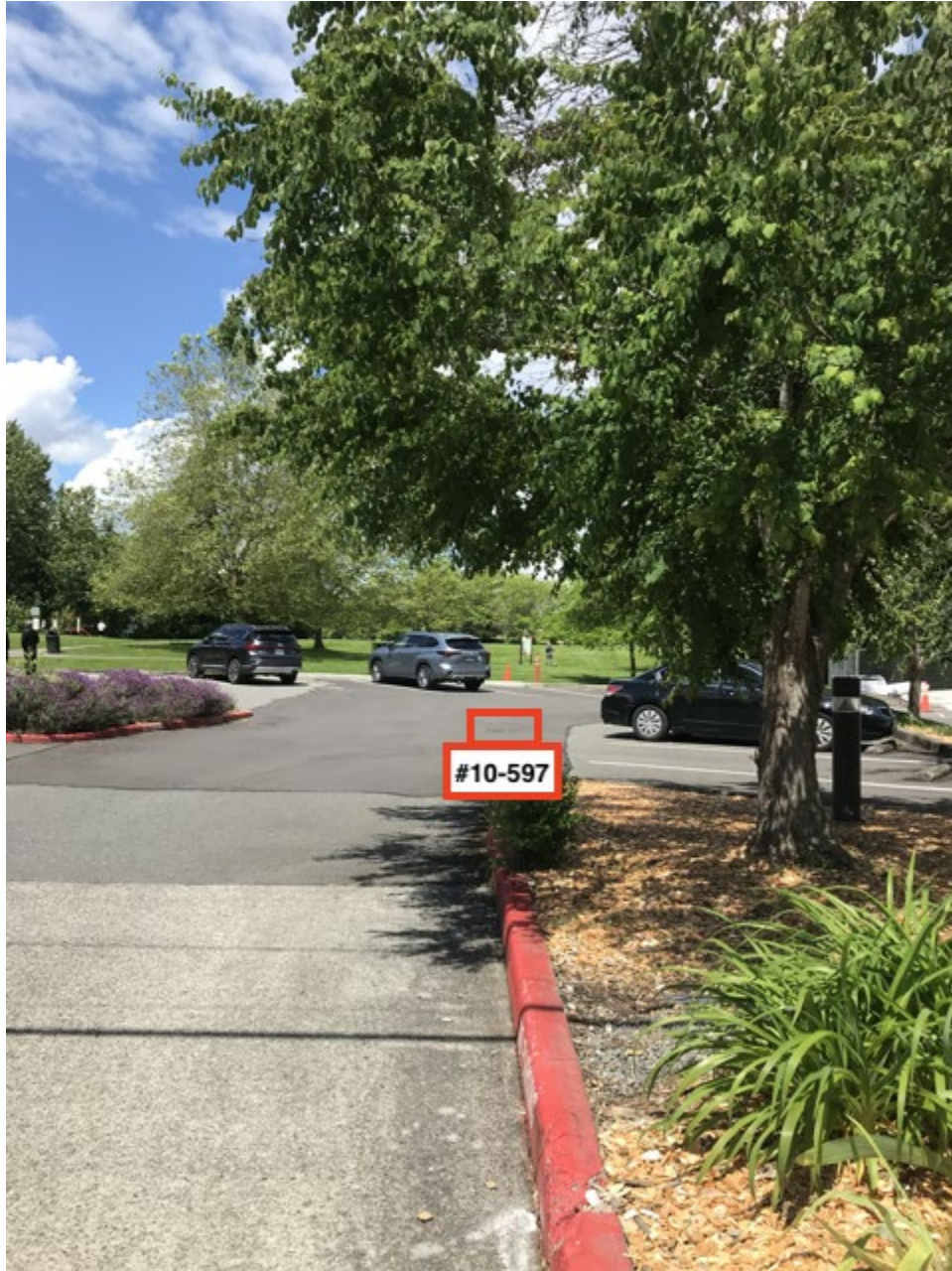
Facing N in the driveway off of SE 34th St entering the parking lot immediately south of Mercedale Park. The location of catch basin #10-597 is marked by a red rectangle.
