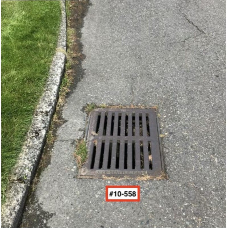
Close up of catch basin #10-558.
